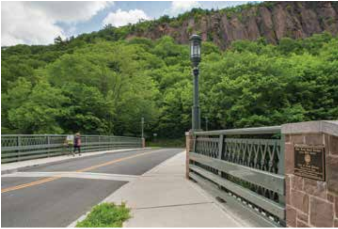
The rehabilitation replicated the ornamental pedestrian rail system and added decorative lighting.
