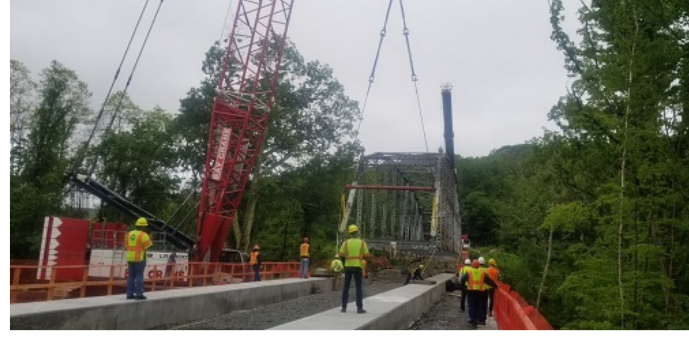
Town Bridge Move - Town of Canton CT/ ROTHA
